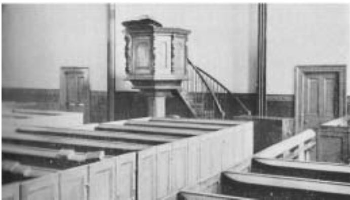
3. The Interior of Shaw Street Chapel.
