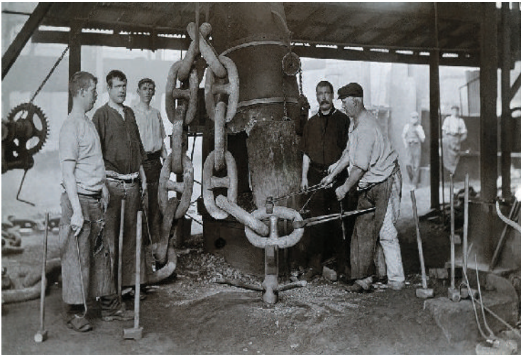
Anchor chain making at the Hingley Ironworks in Netherton, Dudley, which made the anchor and chains for the ill-fated Titanic. Notice the central crossbar through each link for added strength.
